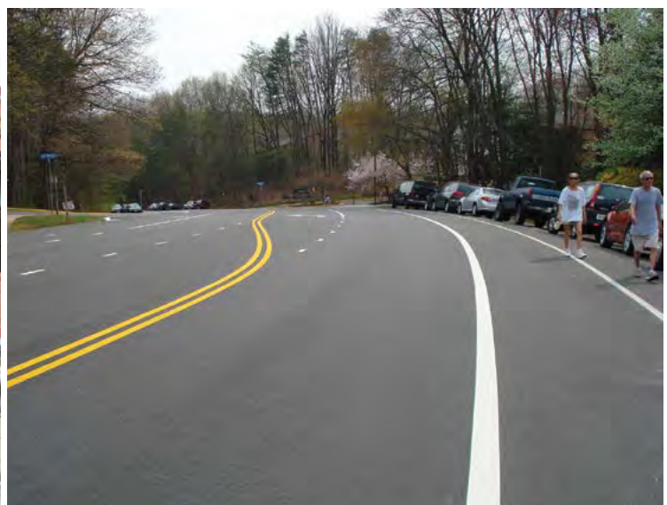
Figure 15. Pedestrians Buffered from Traffic in Reston, VA Photo Credit: Richard Retting
