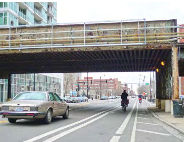
Figure 14. Buffered Bicycle Lanes on Wabash Avenue in Chicago Photo Credit: Stacey Meekins
